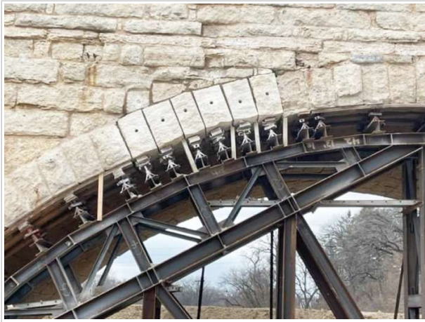
Most of what has been completed on the Keystone Bridge involved what project engineer Nate Miller called “readily visible” tasks, and no visible task has been as significant as the replacement of these six deteriorated stones.
