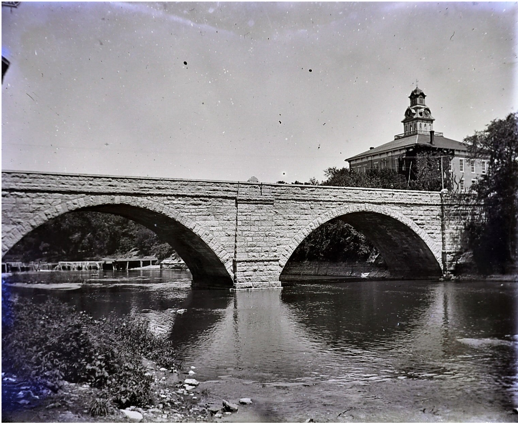
The broken dam dates this photo to late spring 1899. A flood in March of that year destroyed the old John Thompson dam. The Schmidt Brothers rebuilt the dam later that year.
