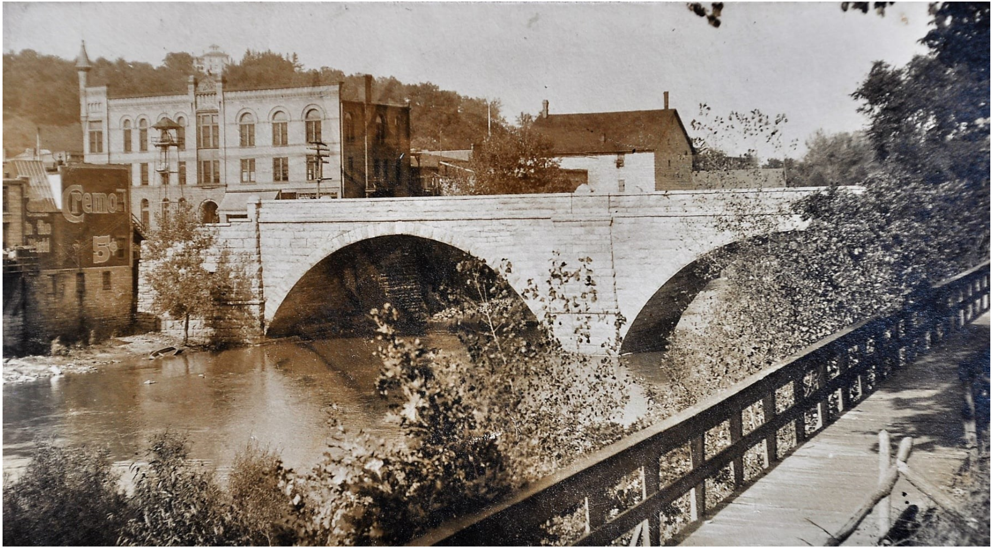
A photo of the bridge with the boardwalk to the train station at the bottom right.
